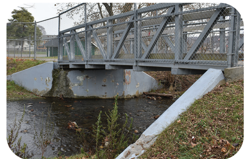
This bridge by the Jr./Sr. High School would be repaired to improve secondary entrance/exit.
